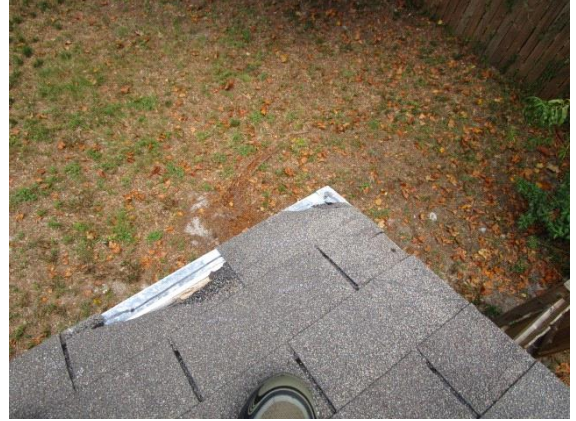
Damaged shingles; exposed sheathing.
