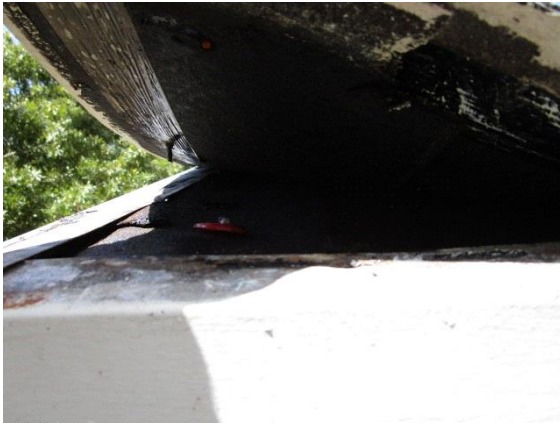
Underlayment under flashing.
