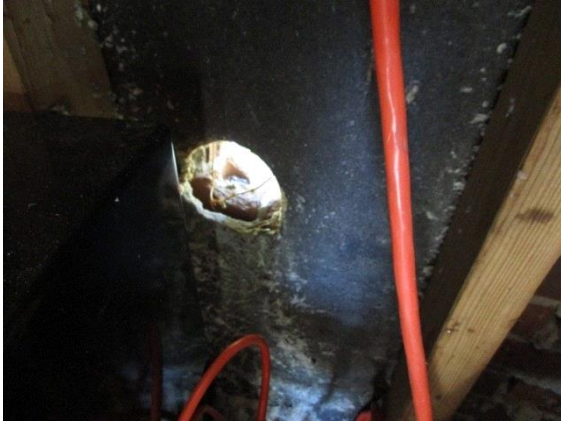
Dryer vent hole from inside.
