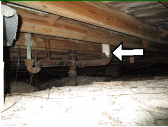
Improper connection.
