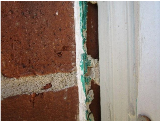
Brick/frame separation.
