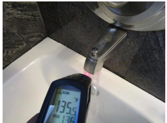
WARNING: Water temp exceedingly hot.
