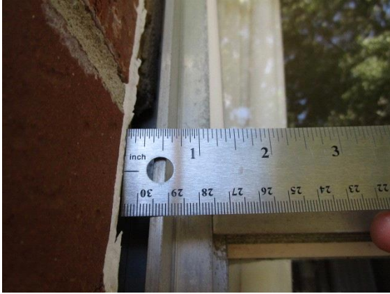
Frame/brick separation
