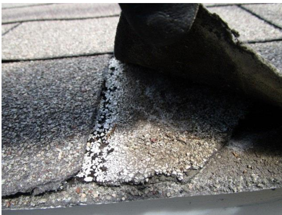
Suspected original roofing under replacement.
