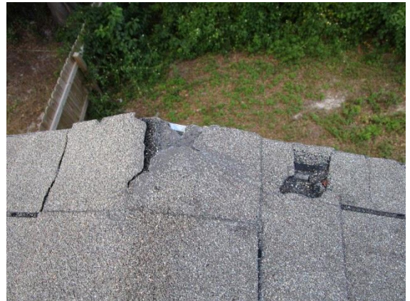
Damaged shingles; exposed sheathing.
